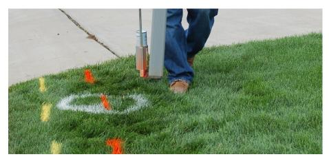
**7.** Structures such as vaults, inlets, and lift stations that are physically larger than obvious surface indications are marked so as to define the parameters of the structure.
